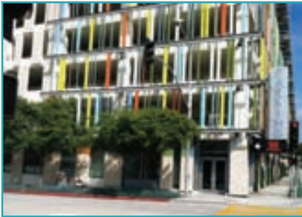
The Civic Center parking structure will accommodate Downtown motorists during construction of Parking Structure 6.
